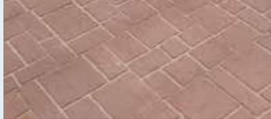
Large format pavers are larger than or equal to 300mm (length) x 300mm (width) and small format pavers are less than 300mm x 300mm. Your choice will depend on the look you wish to achieve.
